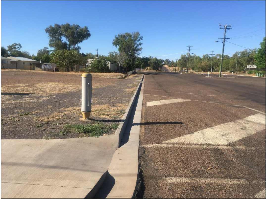
Figure 4—Existing kerb and channel (Source: Developer)
