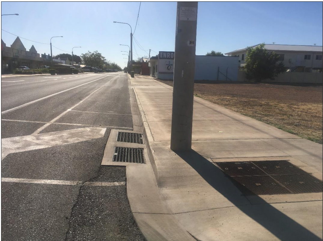
Figure 5—Existing pedestrian linkage (Source: Developer)
