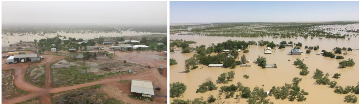
Figure 43: AACo Stations during 2019 flood peak: Canobie (left) and Wondoola (right)
