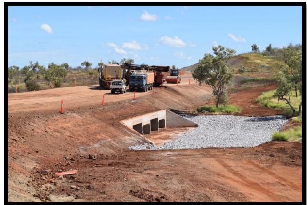
Waste water infrastructure on Andrew Daniels Drive during construction.
