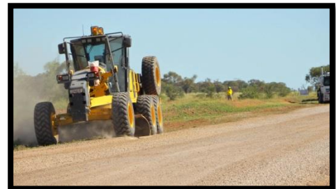
Road formation and sealing on Sedan Dip Road
