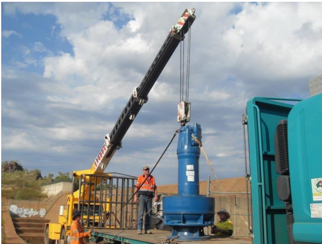
Figure 1 Refurbishment of Harvest Pump at Chinaman Creek Dam
