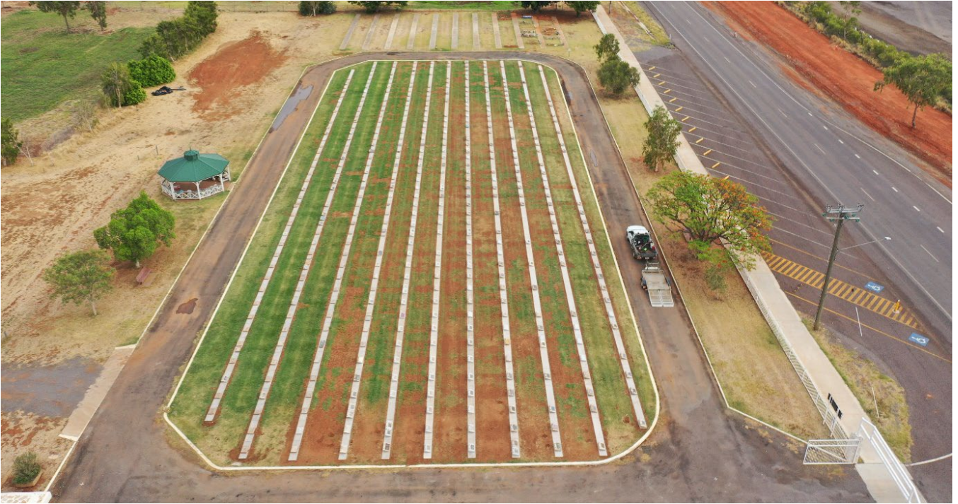
Figure 1: Image showing the recently completed Portion 2 plinths installation.
